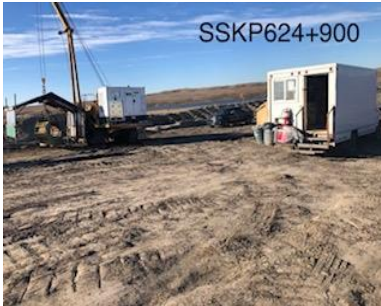
Coating crew mix shack and heater coil shack
