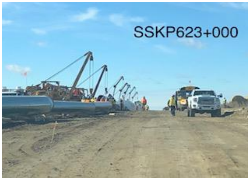
Poor boy welding crew
